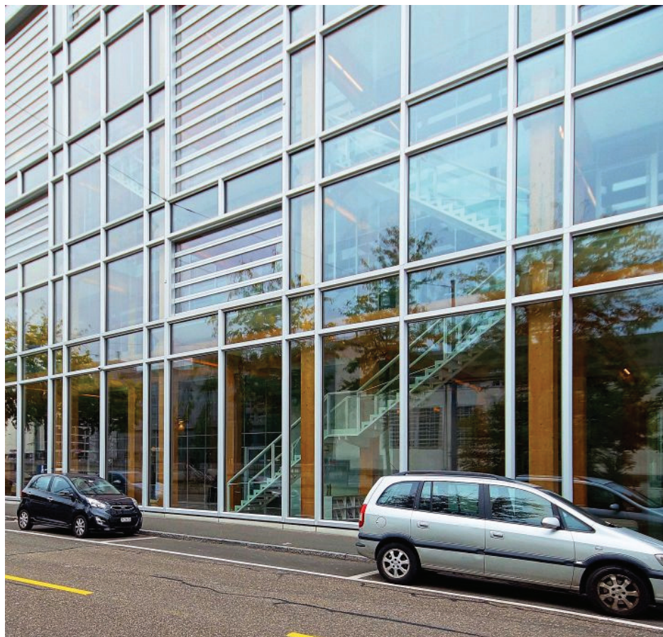
Fig. 2. Tamedia building in Zurich (arch. Shigeru Ban, 2013). Photo by author
