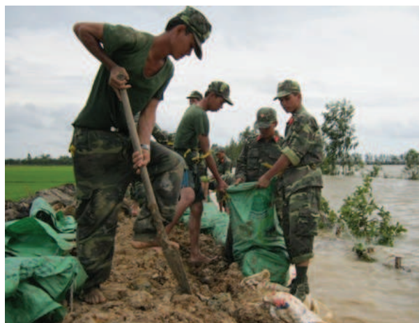
Figure 2. The Army helps the people reinforce the dyke broken in An Giang Province.
