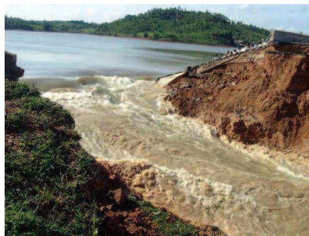
Figure 3. One section of the TAY NGUYEN dam broken in Nghe An and its impact on the surrounding areas.
