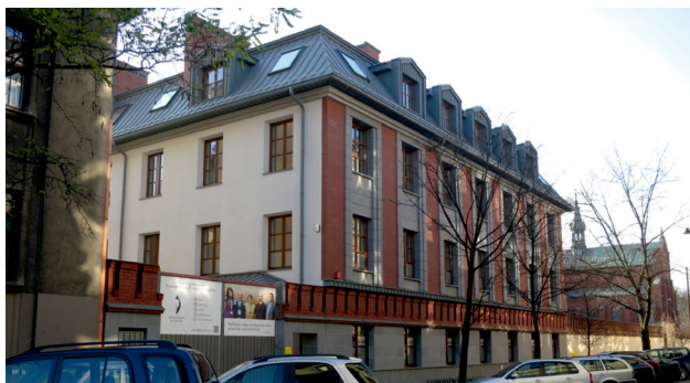
Fig. 2. Building of St. Pio Father Works at Smoleńsk 4 Street in Kraków. Photo by the authors
