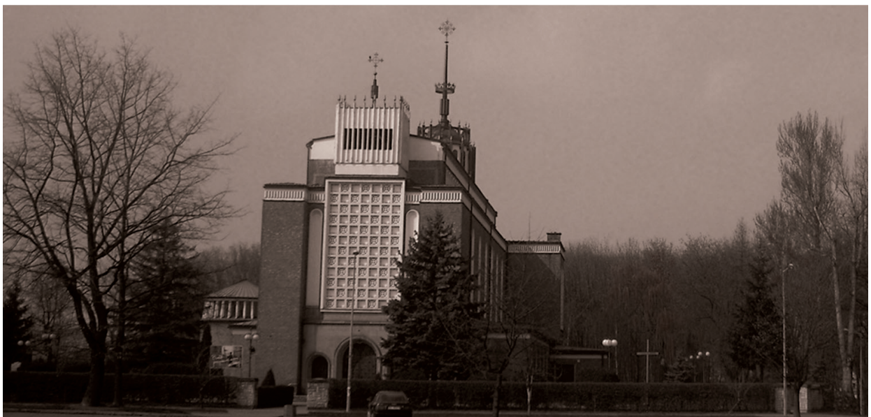
Fig. 5–8. Tarnów-Mościce, Church of Our Lady Queen of Poland, designed in 1941, 1948–1956, by Stanisław Gałęzowski and Władysław Pieńkowski: façade, chancel, side elevation, and view from the square at Topolowa Street. All photos by the authorCCCret
