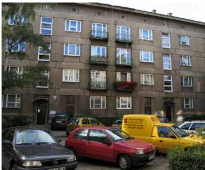
Fig. 3.: "The great slab" - the first realizations following the principles of modernism., One of the first blocks made of Great Slab in Poland. Kraków-Nowa Huta, Hutnicze /Steelworks/ Estate, Mierzwę Street. Realized in 1947.
