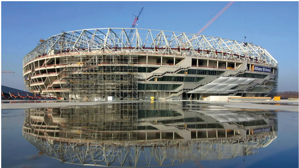
Fig. 2. Allianz Arena in Munich, construction on the stadium (source: [2])
