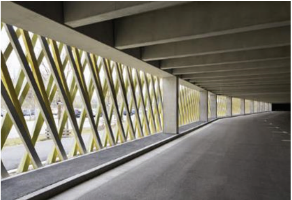
Fig. 15, 16. The view of flood-resistant garage (source: [22])
