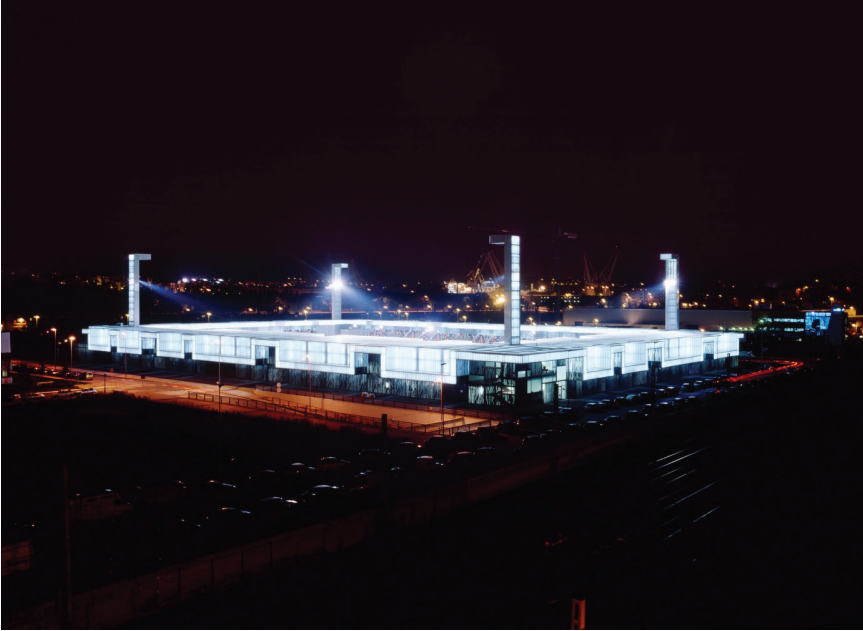
Fig. 9. Lasarre Barakaldo Stadium, Barakaldo, illumination of the stadium during a match, phot. by Roland Halbe (source: [48])
