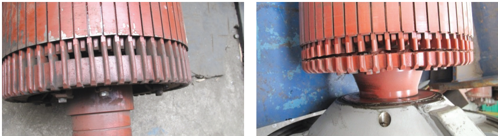
Fig. 6. Junction of rotor winding bars to end-rings: in a brand-new motor (left) and a worn motor with a torn end-ring (right)
