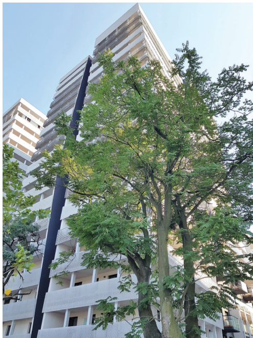
Fig. 5. ATAL Towers – Part II – residential towers, view from the pedestrian promenade
