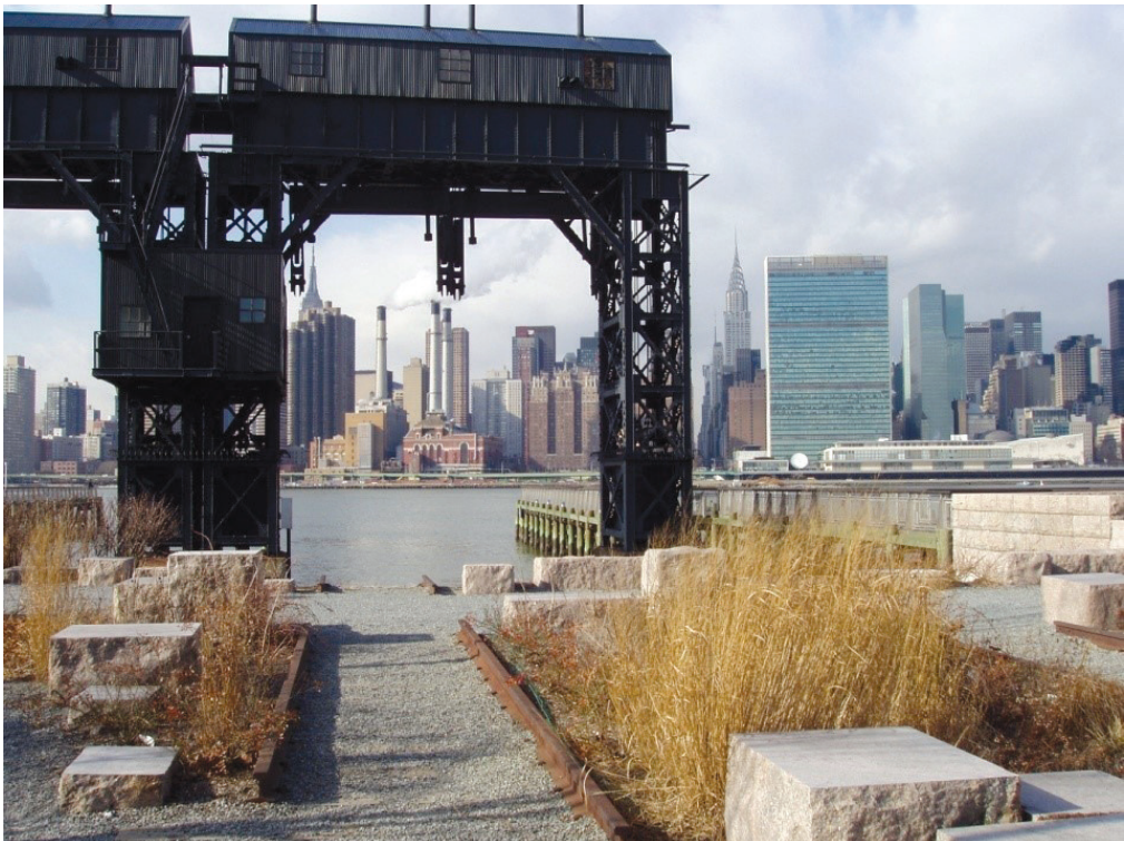
Fig. 5. Historical cranes bearing witness to the area's tradition (photo by W. Gadomska)
