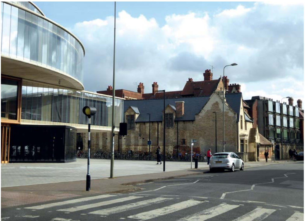
Fig. 13. and 14 Walton Street with the new School set back exposing the sides of neighbouring buildings (photo by I. Samuels)
