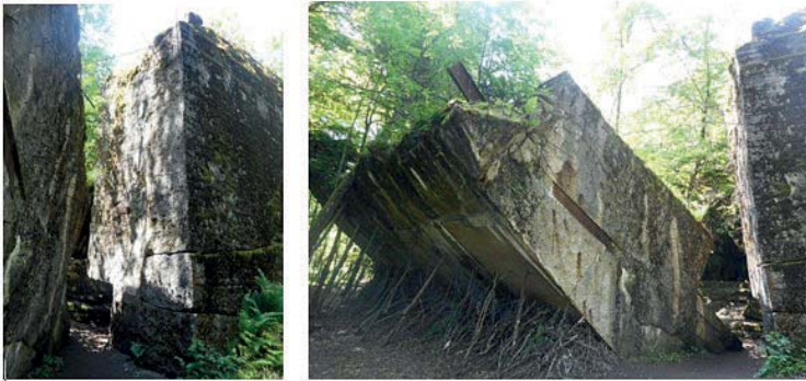
Fig. 13. Concrete wall blocks of heavy bunkers (own photos)
