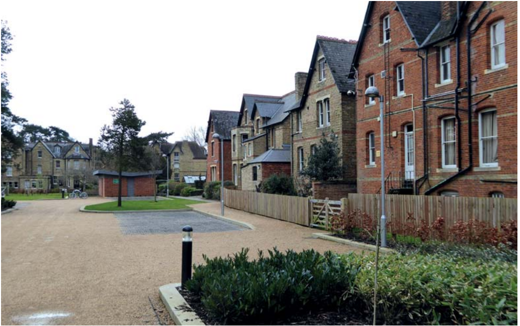
Fig. 11. Private internal street showing access to rear of houses on Canterbury Road (photo by I. Samuels)
