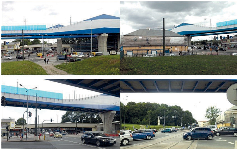
Fig. 7. Views of the Existing State (photos by K. Dudzic-Gyurkovich)
