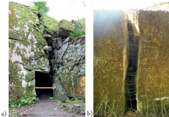
Fig. 14. View of the importance of reinforcement in ensuring ductility and compactness of concrete structures (own photos)
