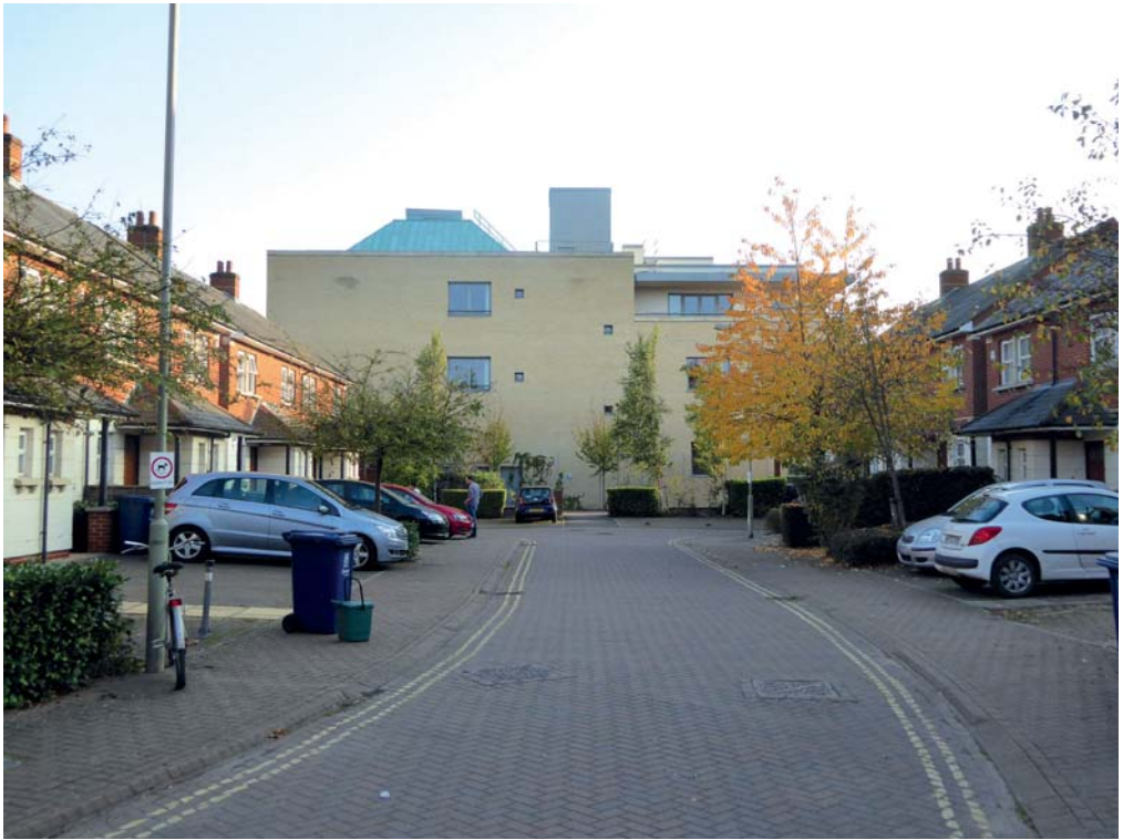
Fig. 17. The north elevation dominating the small scale residential street (photo by I. Samuels)
