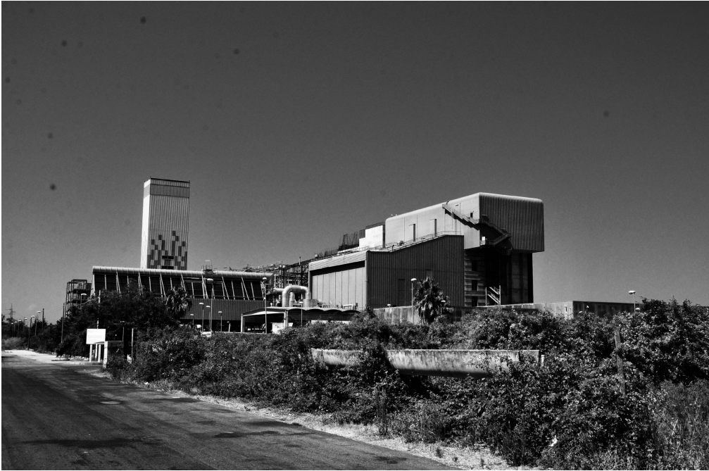
Fig. 2. Eco incineration plant – Gioia Tauro (original work, 2017)
