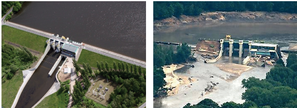
Fig. 7. The Niedów dam and the reservoir of the town of Zgorzelec, before and after the failure
