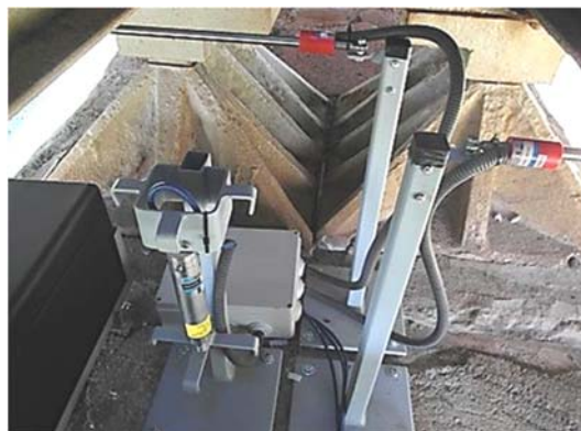
Figure 6. Support structures for mounting angle sensors and displacement sensors at the intermediate support (view on the west side)
