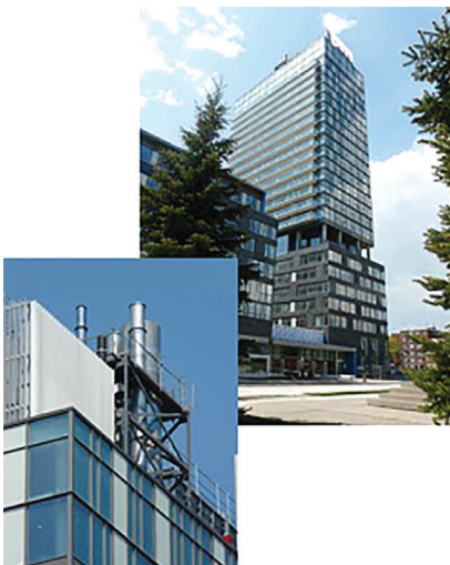
Figs 15 & 16. Regent Park's 22 – story building with district heating plant (inset). Courtesy of Doug Pollard
