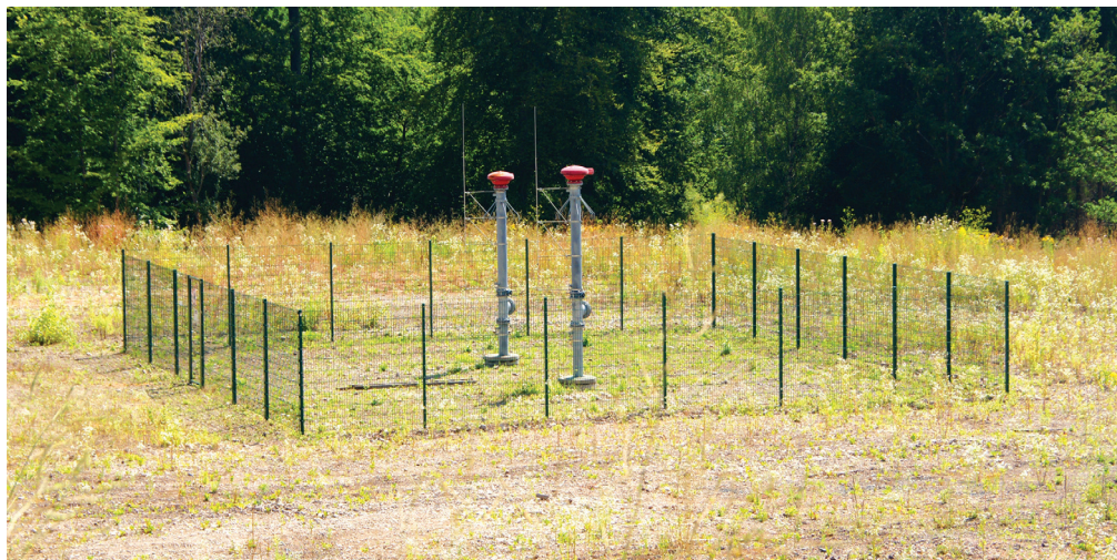
Fig. 3. An installation for degassing liquidated coal workings – the only element marking the former location of mining shaft Lauterbach on the border between Saarland and the Moselle district (photo by P. Langer, 2015)
