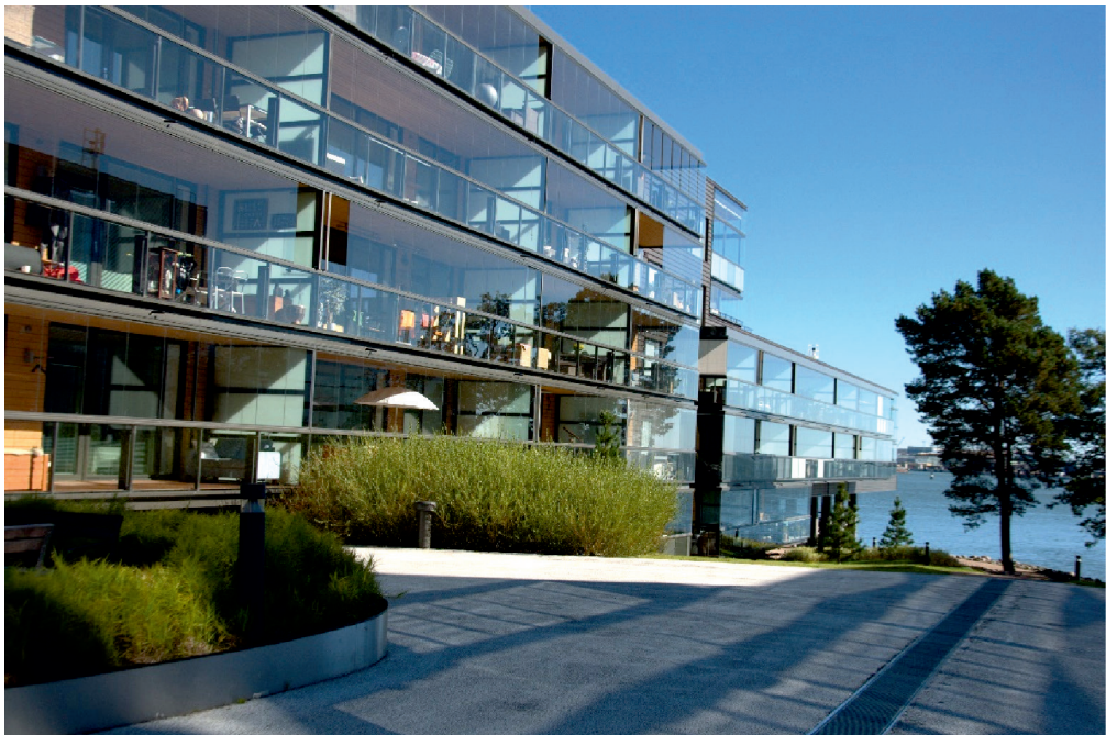
Fig. 5. Residential complex in Lautasaari, Arkkitehdit NRT Oy, Helsinki, 2012 (by the author)
