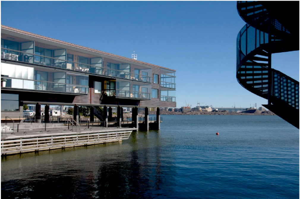
Fig. 6. Residential complex in Lautasaari, Arkkitehdit NRT Oy, Helsinki, 2012 (by the author)
