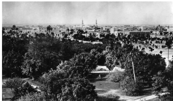
GENERAL VIEW, KHARTOUM (SOUTH WEST)
