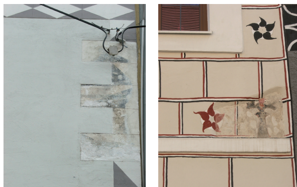
Ill. 10. Original remains incorporated into restored colour schemes: dwellings in Wiener Neustadt (left) and in Görlitz (right). Photos by the author
