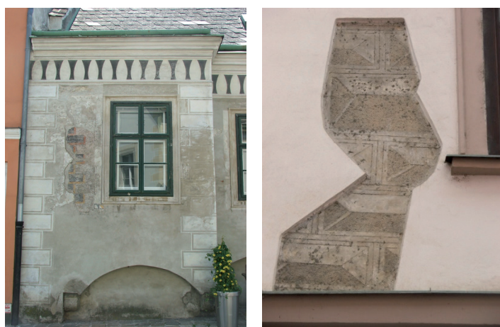
Ill. 9. Traces of historical polychrome on dwelling in Heiligenstadt, Vienna and remains of Renaissance sgraffito in the Old Town in Prague. Photos by the author
