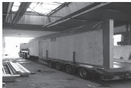
Fig. 2. Loading wall panels onto a vehicle (Nesbau)
