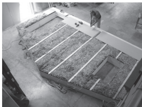
Fig. 6. Prefabricated elements based on wood and straw [9]
