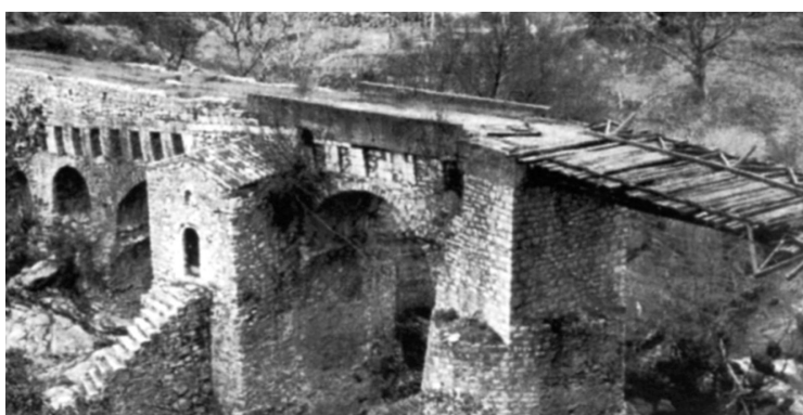
Fig. 7. The medieval bridge in Karytaina (courtesy of G.D. Makris)
