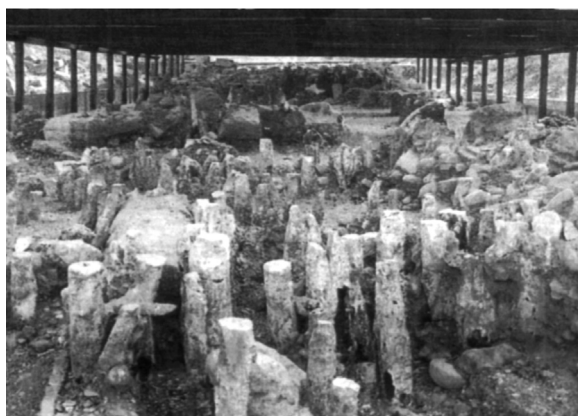
Fig. 3. Wooden piles of the ancient bridge in Amphipolis as they are today (Courtesy of G.D. Makris)
