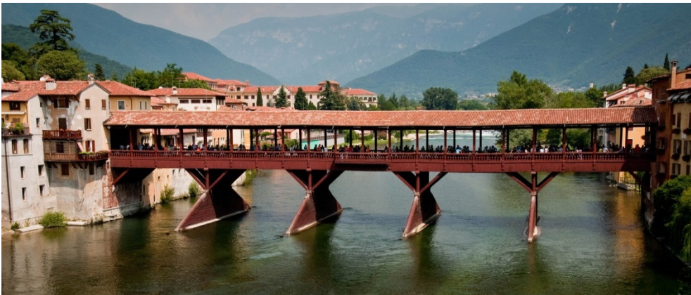
Fig. 10. The current state of a wooden covered bridge Ponte degli Alpini in Bassano del Grappa (source: https://anotherheader.wordpress.com/2010/12/23/italy-bassano-del-grappa , access: April, 2016)
