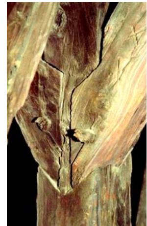
Fig. 7. Assembly marks (photo C.B.)
