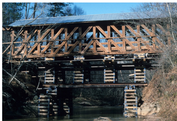
Fig. 15. The heritage Bunker Hill Covered Bridge in North Carolina in the USA with the Haupt's type wooden truss girder (source: http://d.lib.ncsu.edu/collections/catalog/bh0241pnc006 , access: April, 2016)
