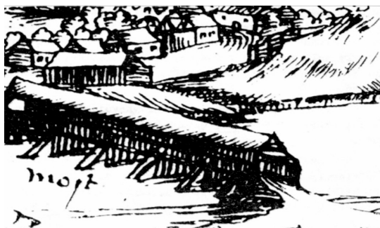
Fig. 9. A covered bridge built in Zvolen over the Hron River, as can be seen in a painting from 1599 made by J. Willenberg (Courtesy of The Monument Boards of The Slovak Republic)
