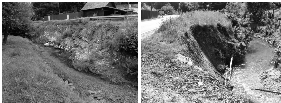
Fig. 1. A damaged fragment of the fill slope and the Prądnik (Białucha) stream undercutting it (Source: [5])
