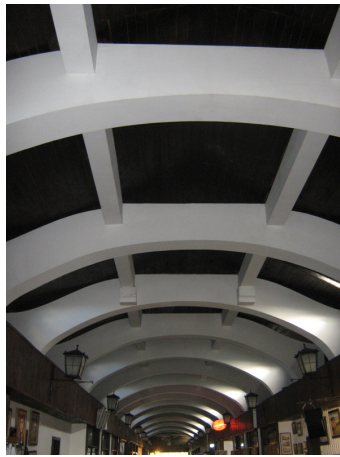
Fig. 9. The ceiling beams in the reconstructed bridge in Lovech (photo by D. Partov, 2013)
