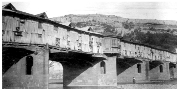
Fig. 5. Views of the old bridge over the Osam River in Lovech (according to [4] – courtesy of N. Tuleskov)
