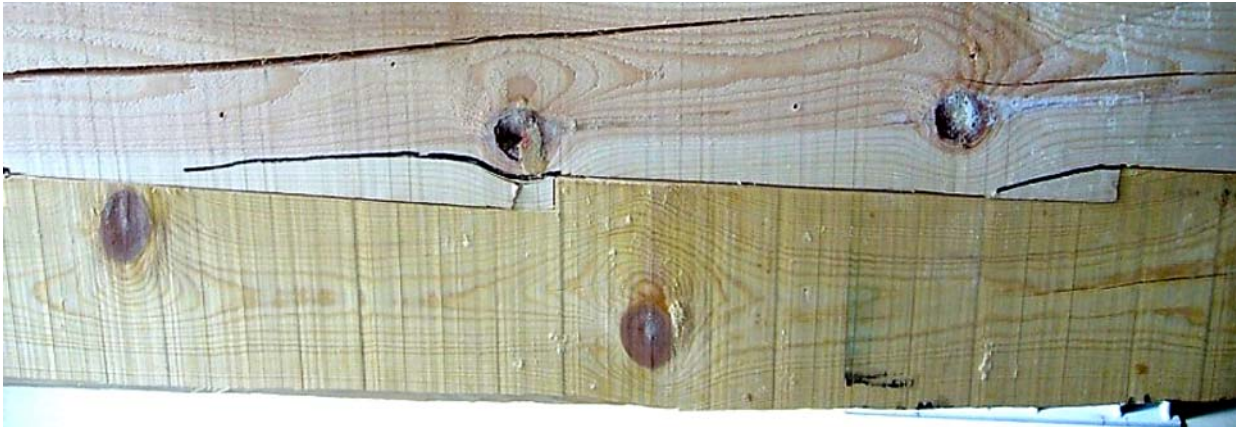
Fig. 14. Specimen 02 – partial fracture in the teathed joints due to knots
