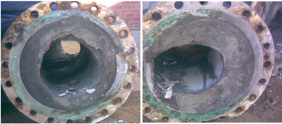
Fig. 1. A view of a pipeline cross-section – the formed scale decreases the free cross sectional area
