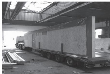
Fig. 2. Loading wall panels onto a vehicle (Nesbau)
