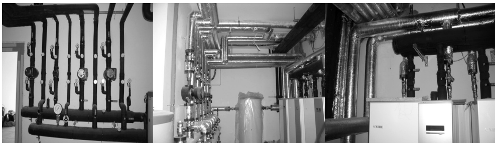
Fig. 2. Heating installations 4 heat pumps brine-water used for heating, ventilation and air-water heat pump for domestic hot water needs
