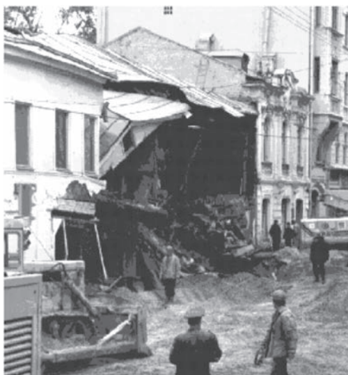
Fig. 4. A building destroyed due to ground uplift from under the foundation to a tunnel executed below, Moscow 1998 [15]
