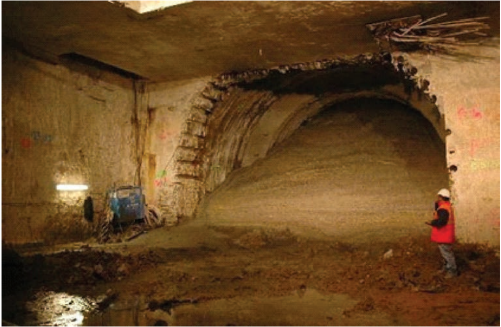
Fig. 5. Initial phase of soil liquefaction after the heave of excavation work ceiling [11]
