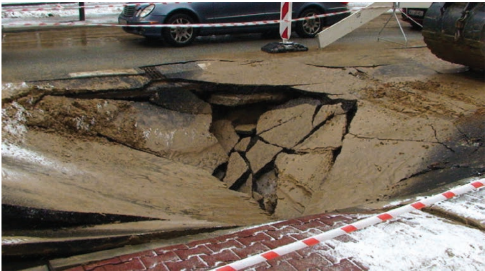
Fig. 3. Subsidence on Koszykowa Street in Warsaw (source: TVN24 publication)
