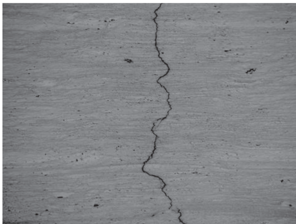
Fig. 2. Crack on the head surface
