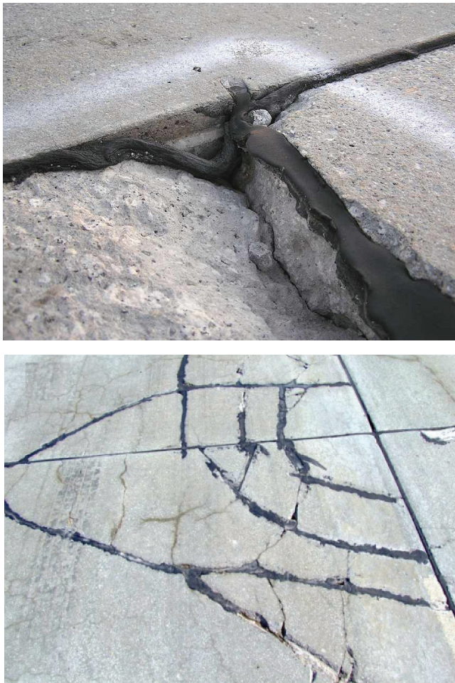
Fig. 1. Damaged expansion gap filled with bitumen
