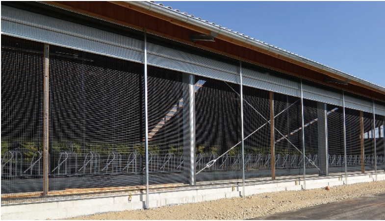
Fig. 1. A utility building with openwork side walls
