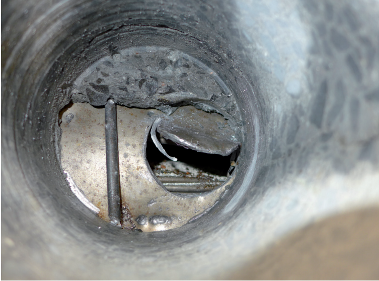
Fig. 4. View into the drilled hole in the girder subjected to investigation. The steel cover of the prestressing cable duct and its interior are visible
