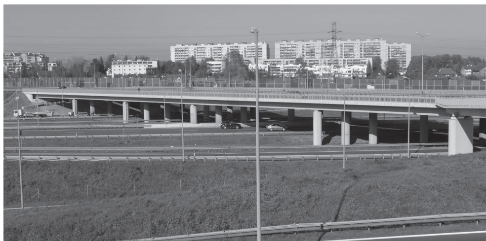
Fig. 1. View of the structure
