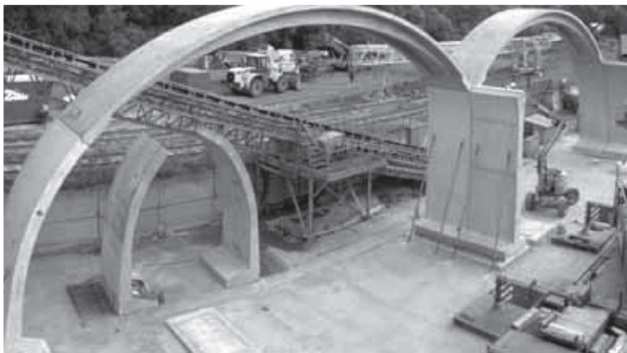
Fig. 2. Construction of the arch of Matiere system made of prefabricated elements
