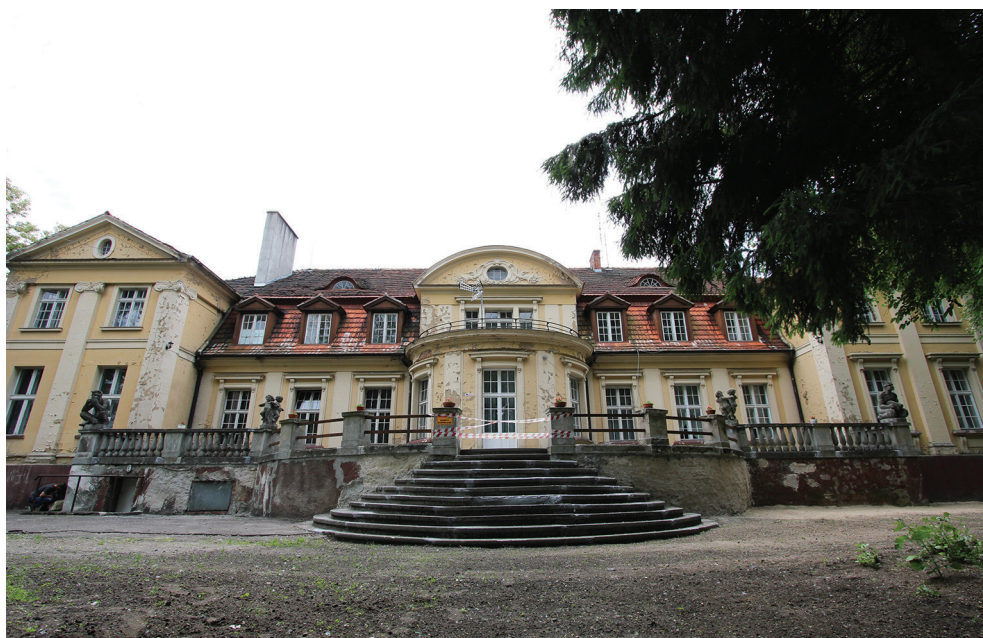
III. 2. Pałace in Bieganowo, garden elevation with a terrace, current condition (photo by J. Białkiewicz)
