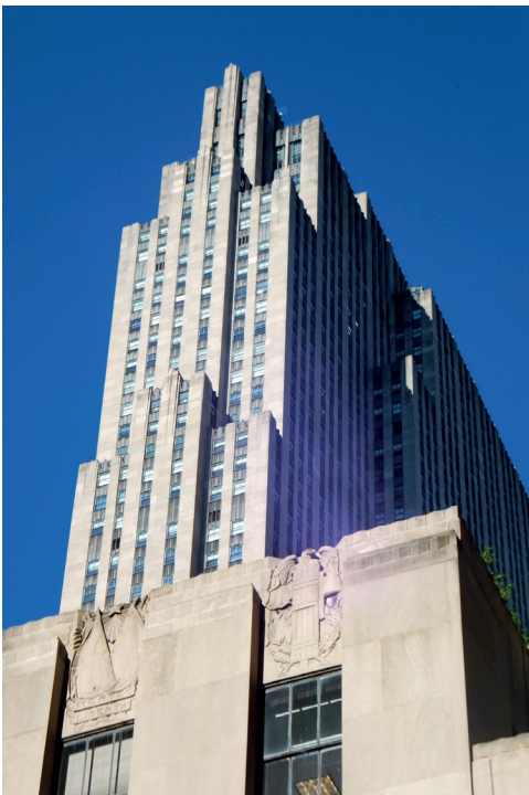
III. 3. GE Building (RCA Building or 30 Rock), Leading architect – Raymond Hood (photo by author, New York 2014)
