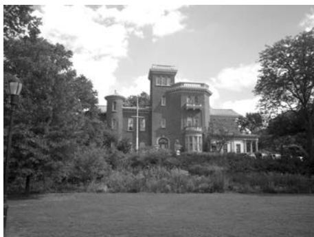
III. 11. Lighfield Villa (photo by author 2014)
