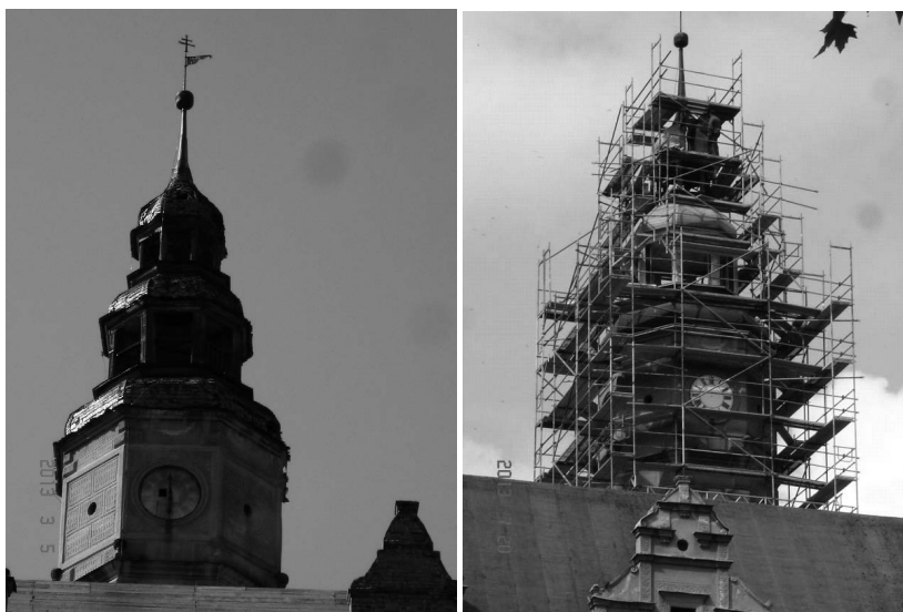
Fig. 4. View of the clock tower. On the left before renovation, to the right during the renovation
