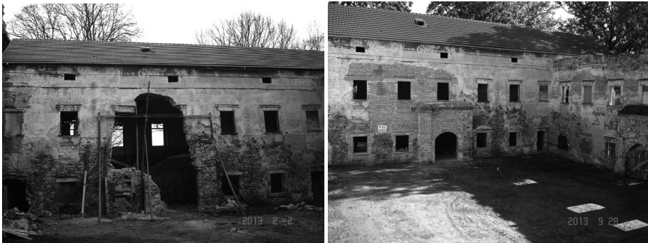
Fig. 2. View of the administration wing and repairs which have been made using ceramic brick. Left side is a view on the day of February 2nd, 2013 to the right as at September 28th, 2013
