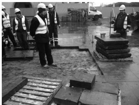
Fig. 4. Methods of dismantling stone slabs: a) Manual b) Mechanical (source: Royal Castle on Wawel Hill archives)
