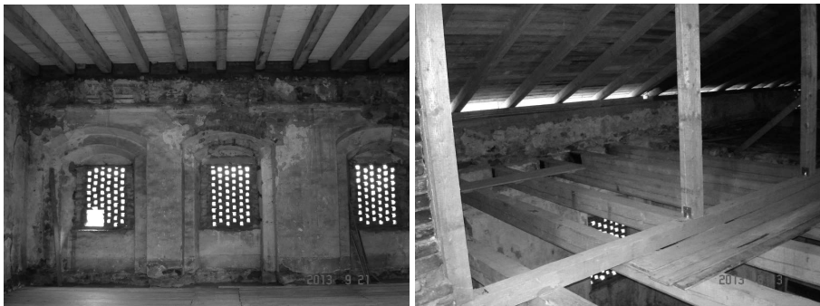
Fig. 3. Wooden beam-framed floors restored in the north wing of the palace
