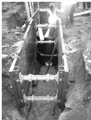
Fig. 2. Method of securing excavation walls: a) for reopened excavations b) for new excavations, with prior archaeological reconnaissance (source: Royal Castle on Wawel Hill archives)
