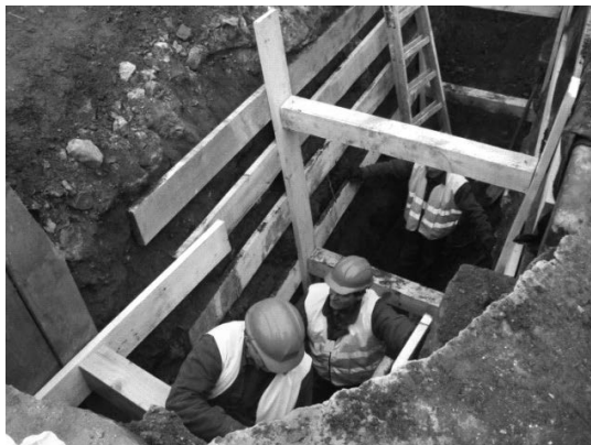
Fig. 2. Method of securing excavation walls: a) for reopened excavations b) for new excavations, with prior archaeological reconnaissance (source: Royal Castle on Wawel Hill archives)
