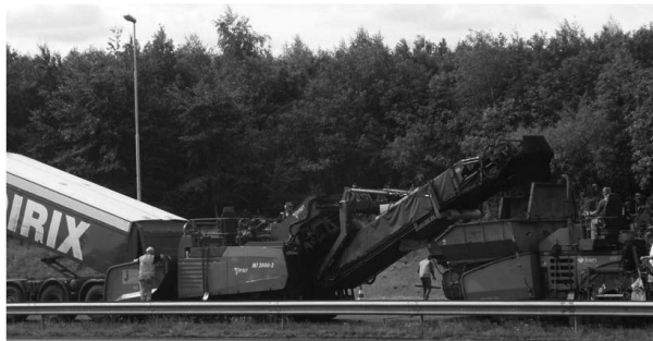
Fig. 7. Resurfacing: machine set of paver, feeder and truck at work (2013) (source: Z. Tokarski)
