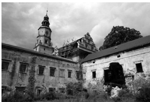
Fig. 1. View of the facade and roofing in the east wing, on the day of August, 2011 [2]
