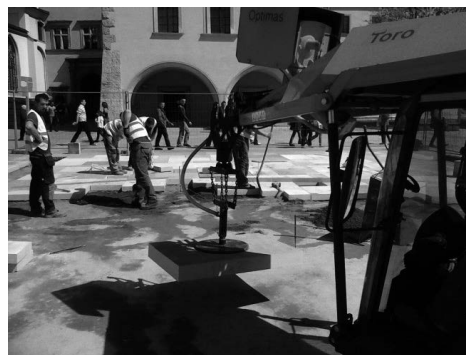
Fig. 4. Methods of dismantling stone slabs: a) Manual b) Mechanical (source: Royal Castle on Wawel Hill archives)
