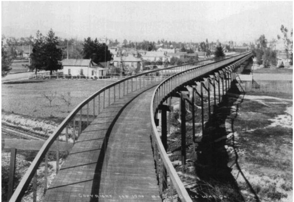
Ill. 6. A tolled elevated cycleway connecting Pasadena and South Pasadena in 1900 (Dobbins Collection, Pasadena Museum of History)
