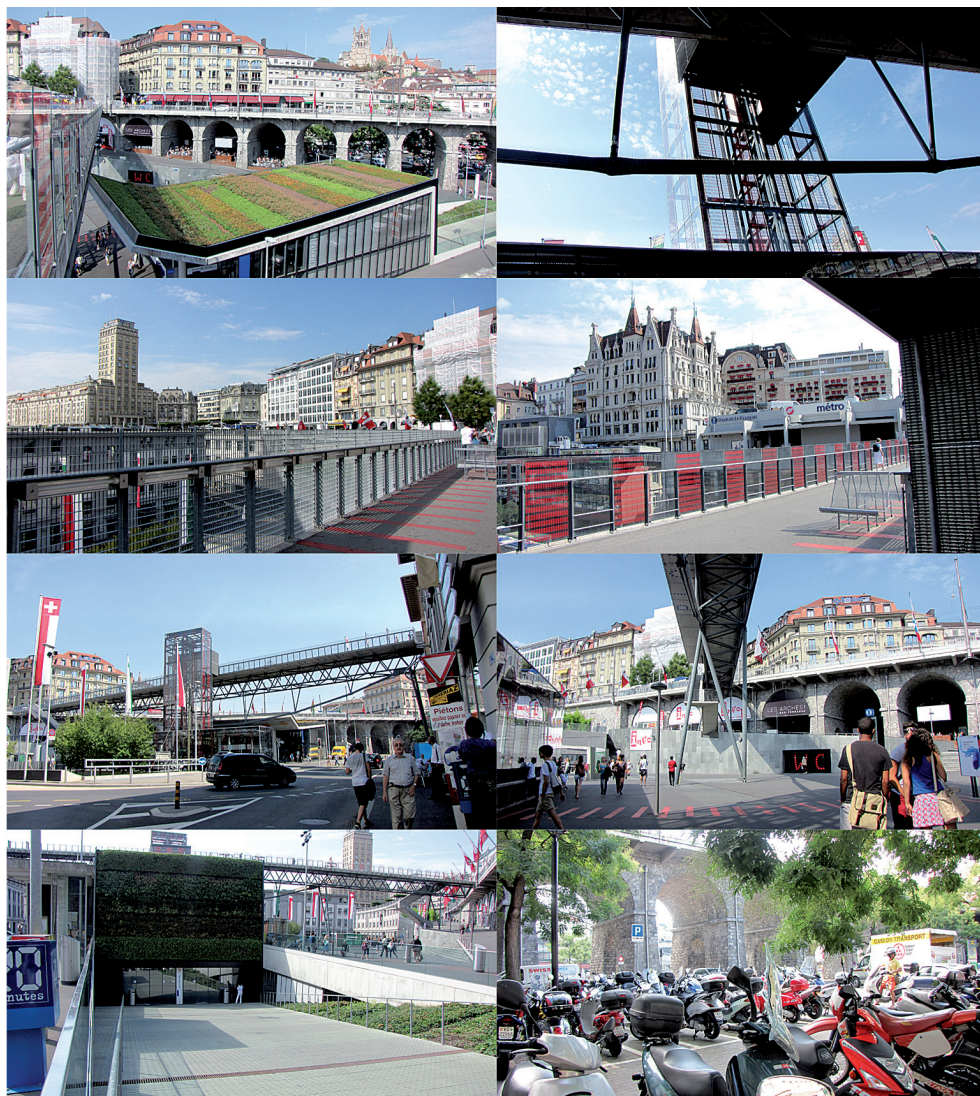
III. 5. Redevelopment of Place d'Europe, Bernard Tschumi, M+V, 1994–2001
