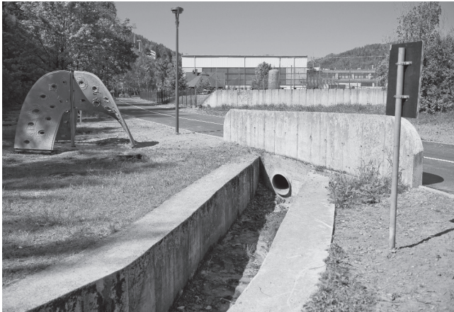
III. 5. Unprotected infrastructure elements next to a playground (photo by the author, 2012)
