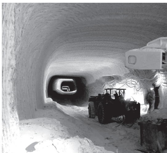
Ill. 7. Bare (i.e. with no lining) corridor working pit drilled in the rock salt deposit “Kazimierzów” within the area of the KGHM mine “Polkowice-Sieroszowice” (photo by the author)
