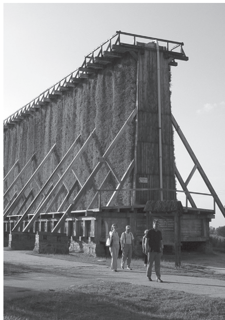
Ill. 4. Brine graduation tower in Ciechocinek built in the 20s of the 19 th century for the needs of the local pan brine boiling plant (photo by the author)
