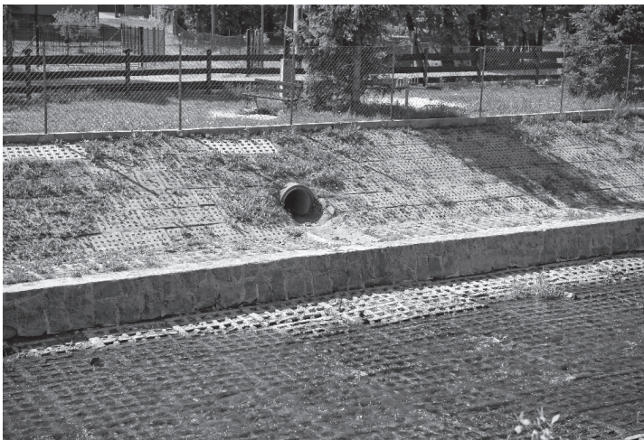
III. 9. One of the storm water drainage outlets (photo by the author, 2012)
