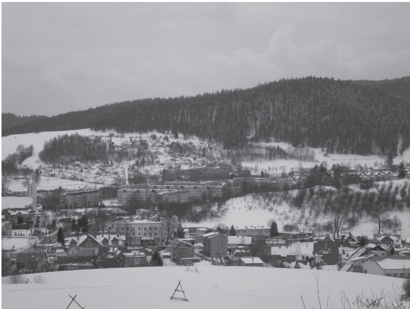
Ill. 2. Krynica, multi-family development in Czarny Potok. The layout and architectural form do not comply with the local conditions (photo by the author, 2012)
