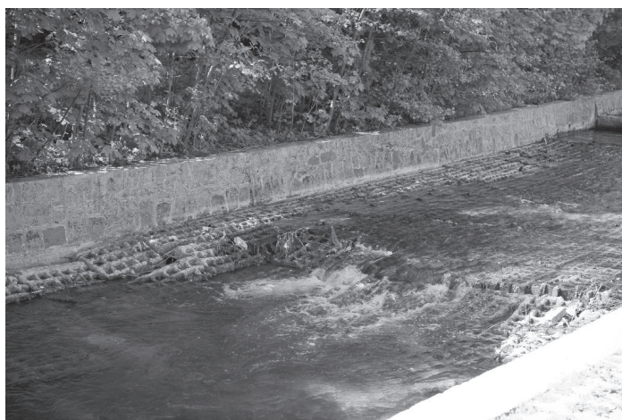
Ill. 7. Damages to the artificial riverbed bottom (photo by the author, 2012)
