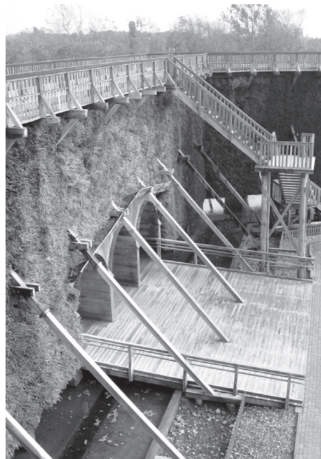
Ill. 5. The structure of the historic-value brine graduation tower in the area of the spa resort park in Inowroclaw is this right? (photo by the author)
