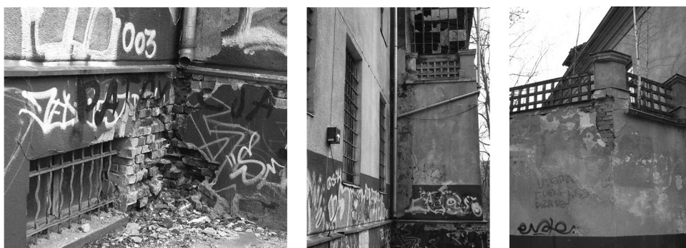
Fig. 14–16. The damage to walls caused by soaking, 2008
