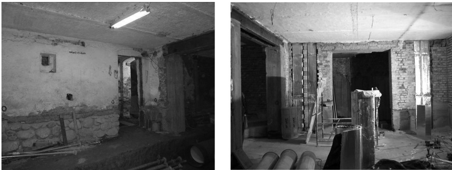
Fig. 21, 22. The works of deepening the cellar, 2011
