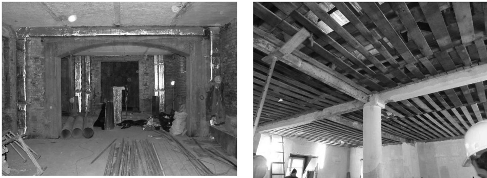
Fig. 4, 5. The brick ceiling above the basement and the timber ceiling (above the attic) supported by steel binding joists and a steel column, 2011
