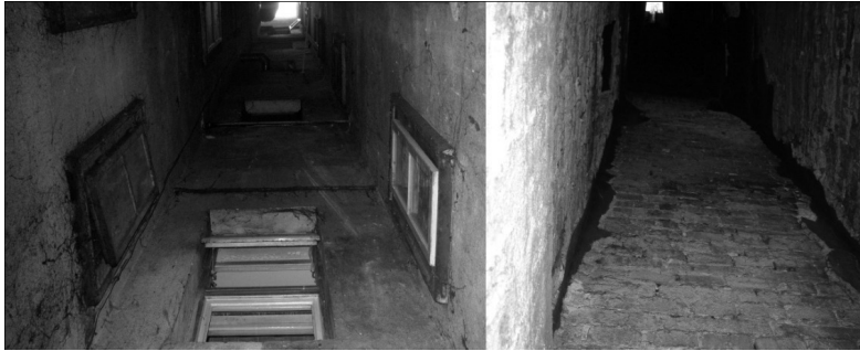
Fig. 3. Interior view of the air-shafts
