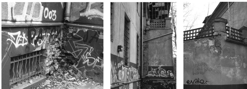
Fig. 14–16. The damage to walls caused by soaking, 2008
