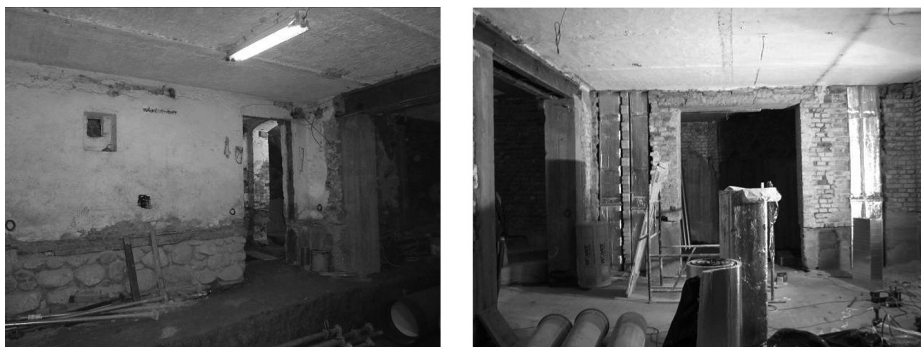
Fig. 21, 22. The works of deepening the cellar, 2011
