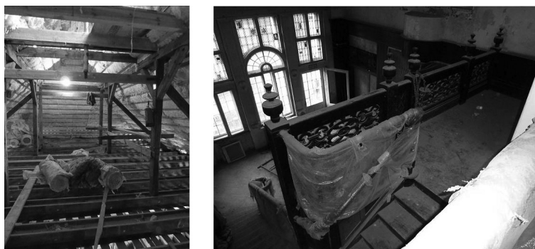
Fig. 8, 9. The timber roof structure and the view from the entresol over the two-storey fireplace ballroom with stained glass windows, 2011
