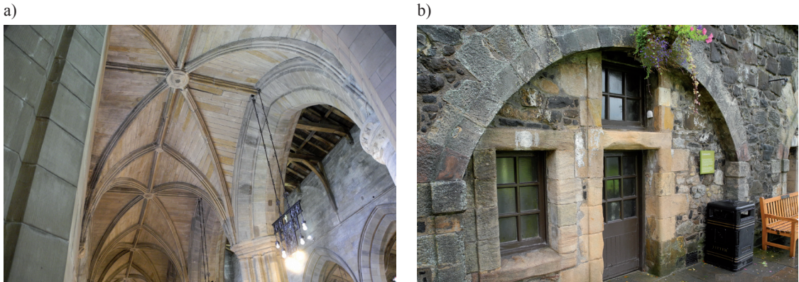
III. 2. a) A stone star-vault in the Church of the Holy Rude (1440–1480) and b) Stone portal of the entrance in the Stirling Castle (Scotland)
