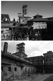
Fig. 3. “Julia” mine in Wałbrzych – condition of buildings before renovation [9]
