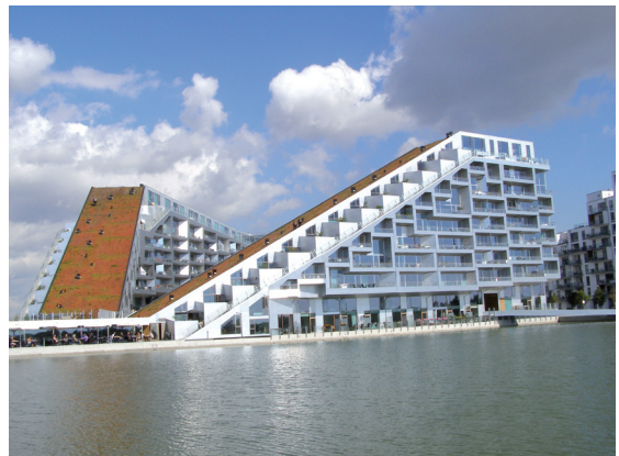
III. 12. Copenhagen – Ørestad. 8 House (Danish: 8 Tallet) designed by Bjarke Ingels Group (author's photo)
