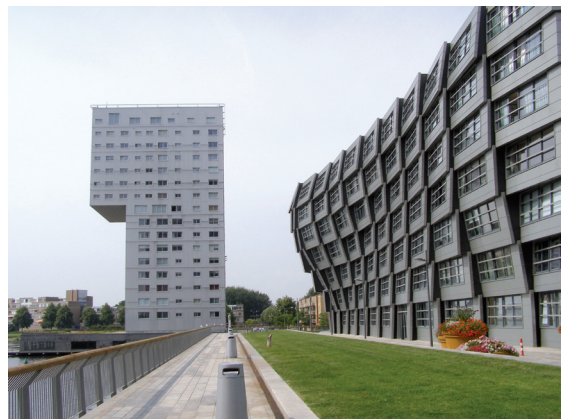
III. 9. Almere – the Wave (building), arch. René van Zuuk; in the distance Silverline designed by Claus en Kaan Architecten (author's photo)
