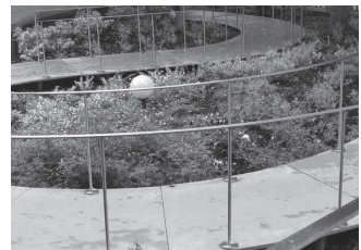
III. 14. Application of RPC (Reactive Powder Concrete) – “Ductal®”: pathway – “Flying Carpet”, Tomi Ungerer Museum – International Centre for Illustration, Strasbourg, France, 2007 [52]
