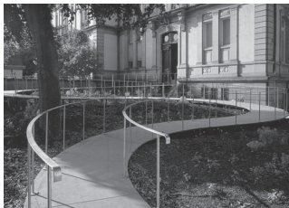
III. 14. Application of RPC (Reactive Powder Concrete) – “Ductal®”: pathway – “Flying Carpet”, Tomi Ungerer Museum – International Centre for Illustration, Strasbourg, France, 2007 [52]
