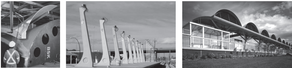
III. 7. Application of RPC (Reactive Powder Concrete) – “Ductal®”: Shawnessy Light Rail Train (LRT) Station (RPC precast elements: ultra-thin (2 cm) curved roof shell, columns), Calgary, Canada, 2004 [40]
