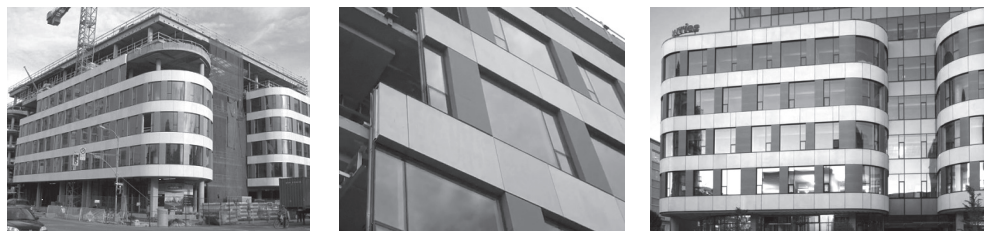
III. 10. Application of RPC (Reactive Powder Concrete) – “Ductal®”: façade panels (curtain wall system) (ultra-thin), “The Atrium”, Victoria, Canada, 2010 [12, 52]
