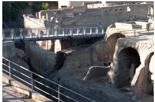
III. 17. Herculaneum – suspension bridge over excavations
