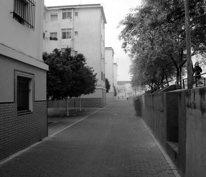
il. 4. Existing slope due to old defence wall. Source: Authors
