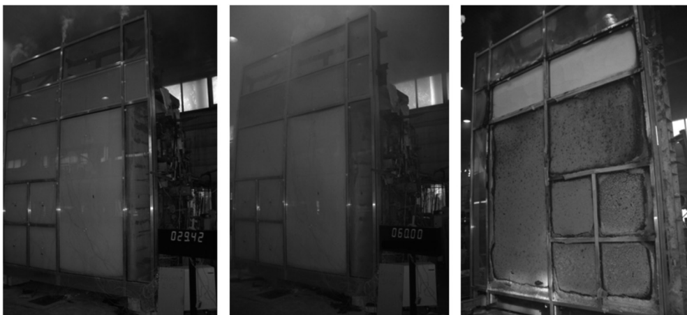
III. 2. The impact of fire on the curtain wall, visible movement of hot air and gases inside the carrier profiles (source: B. Sędlak, Fire resistance tests of glass curtain walls , part 2, in Świat Szkła (The World of Glass) 10/2012)
