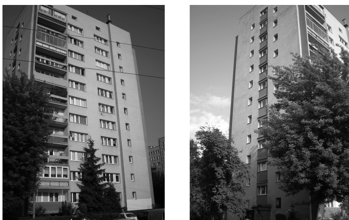
Fig. 1. North and East elevations of analyzed building
