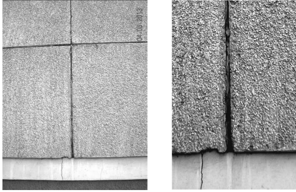
Fig. 2. Panel connection joint – external view
