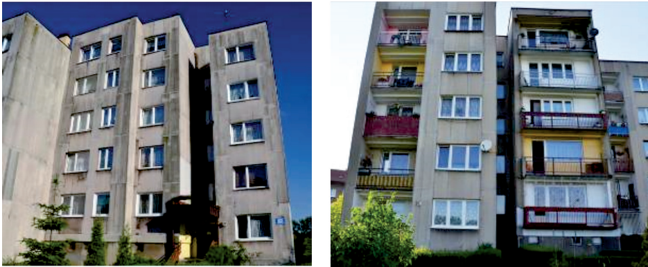
Fig. 1, 2. Bytom, view of the surveyed building, north-west elevation (1) and south-east elevation (2)
