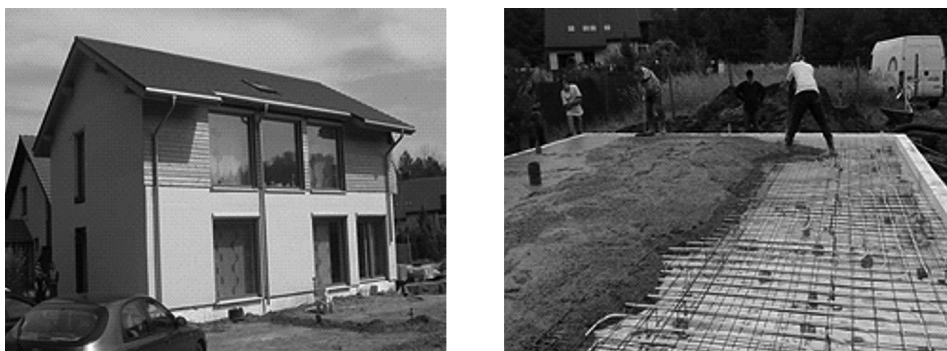
Fig. 1. Passive house in Boruszowice (left) and slab on grade during construction (right)
