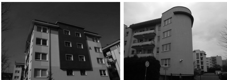
Fig. 1. Examples of building facades erected after 2000
